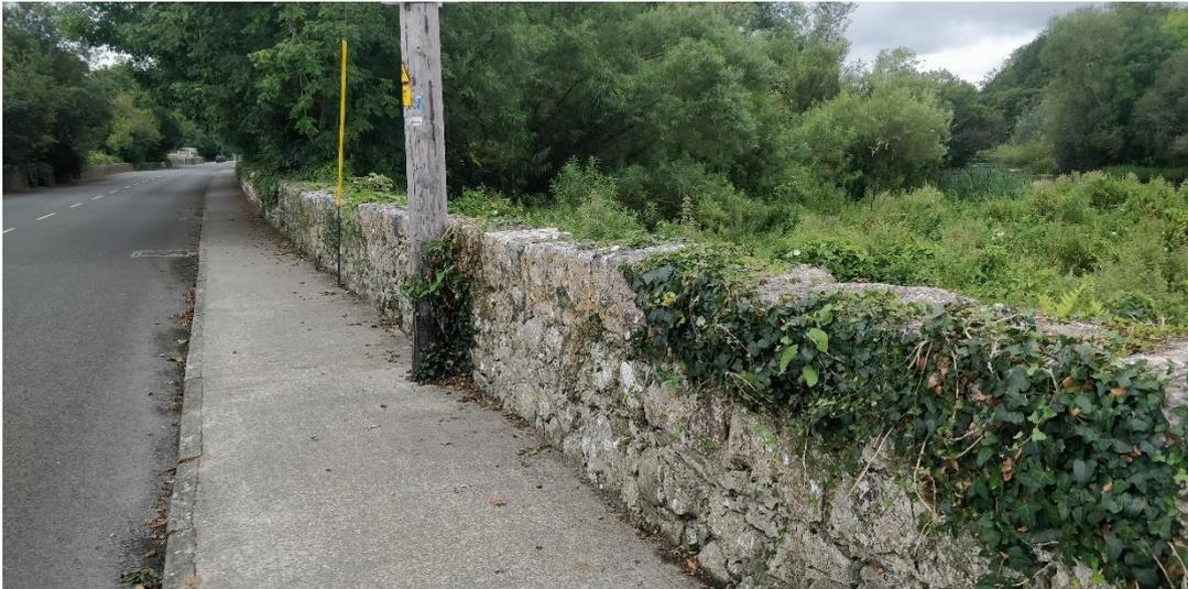
**Figure 8-16: Mall road wall, which will be demolished and stone re-used in construction of new flood wall**
