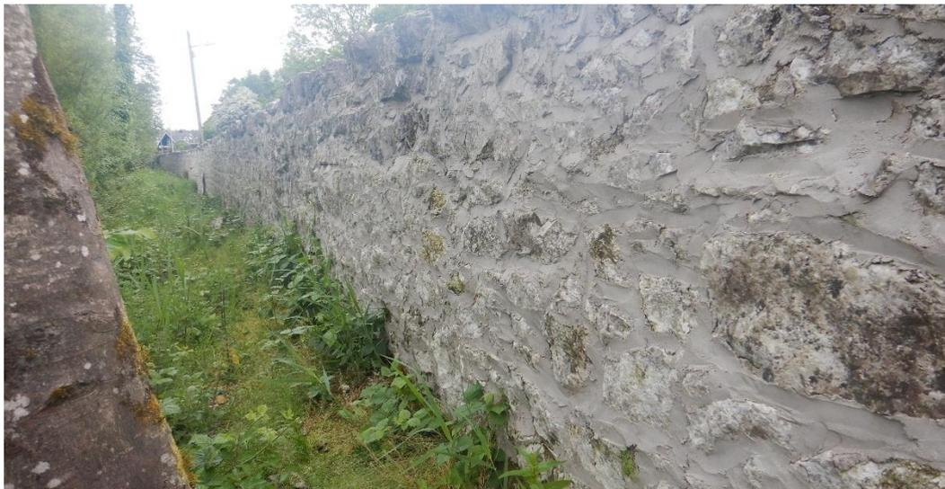
**Figure 8-17: River side of Mall road wall, recently re-pointed**
