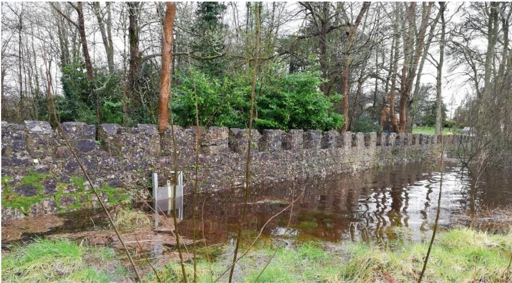
**Figure 8-44: Three sluices at Island House Causeway, shut during winter flooding**
